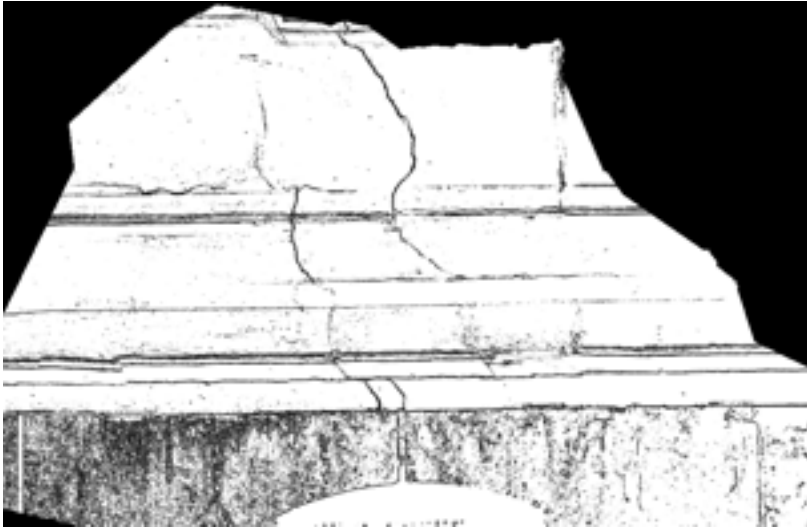
C) Processed image as texture on 3D photogrammetric model
