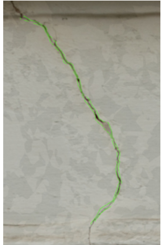
D) Polyline (in green) traced along crack edges on photorealistic texture
